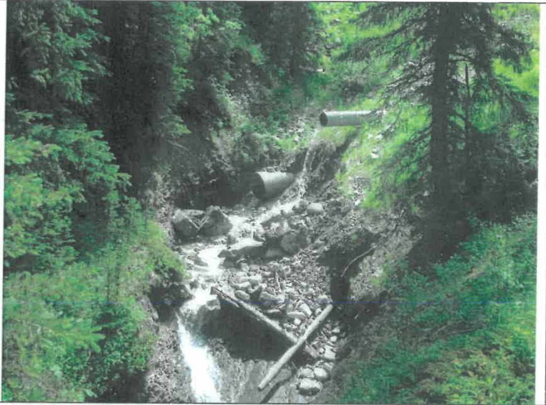
Downstream (east) end.
