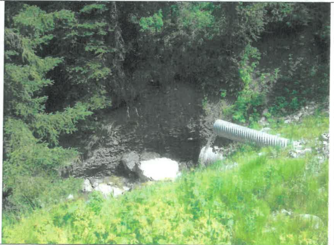
Downstream (east) end.
