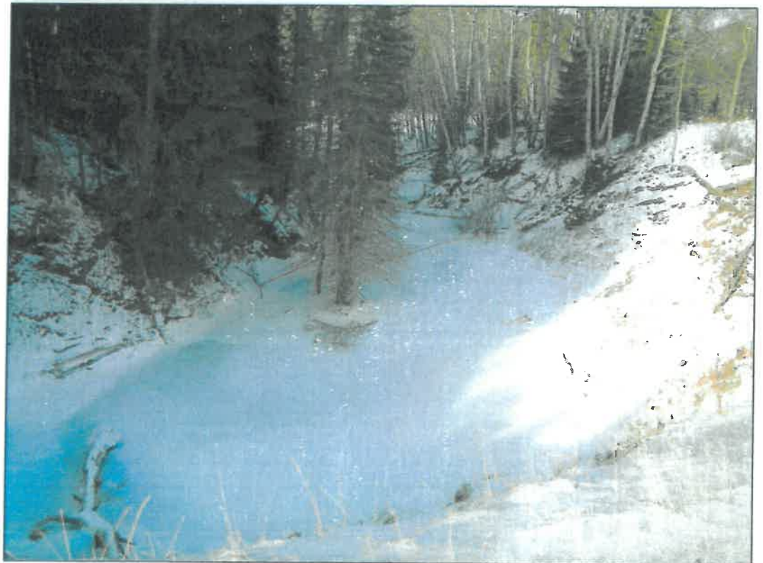
Looking Upstream (west) from roadway at backwater created by drift blockage.
