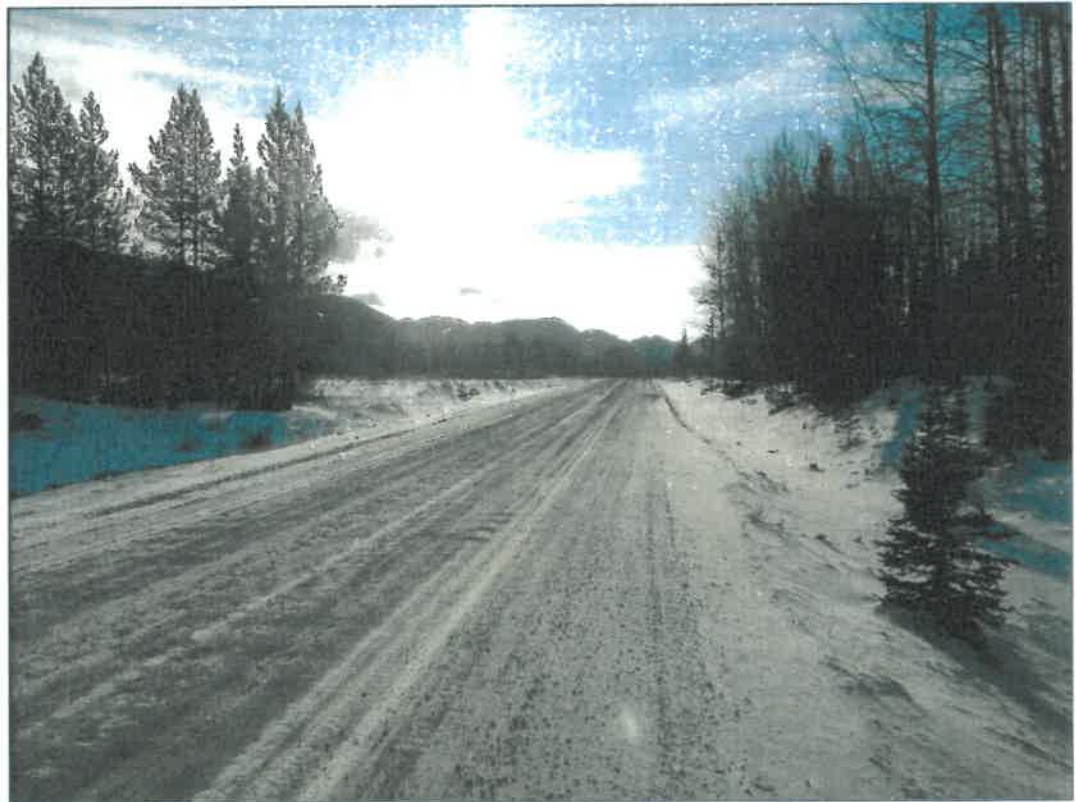
Looking South at approach road over crossing.
