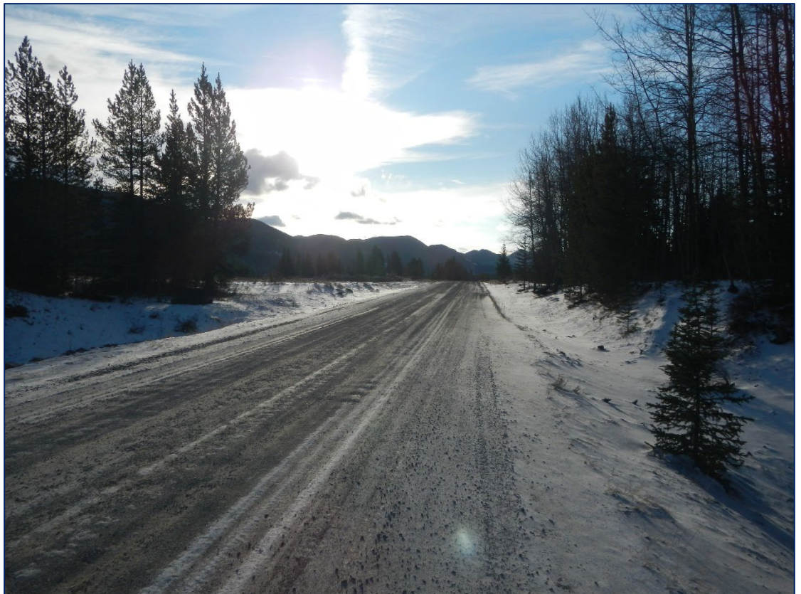
Looking South at approach road over crossing.
