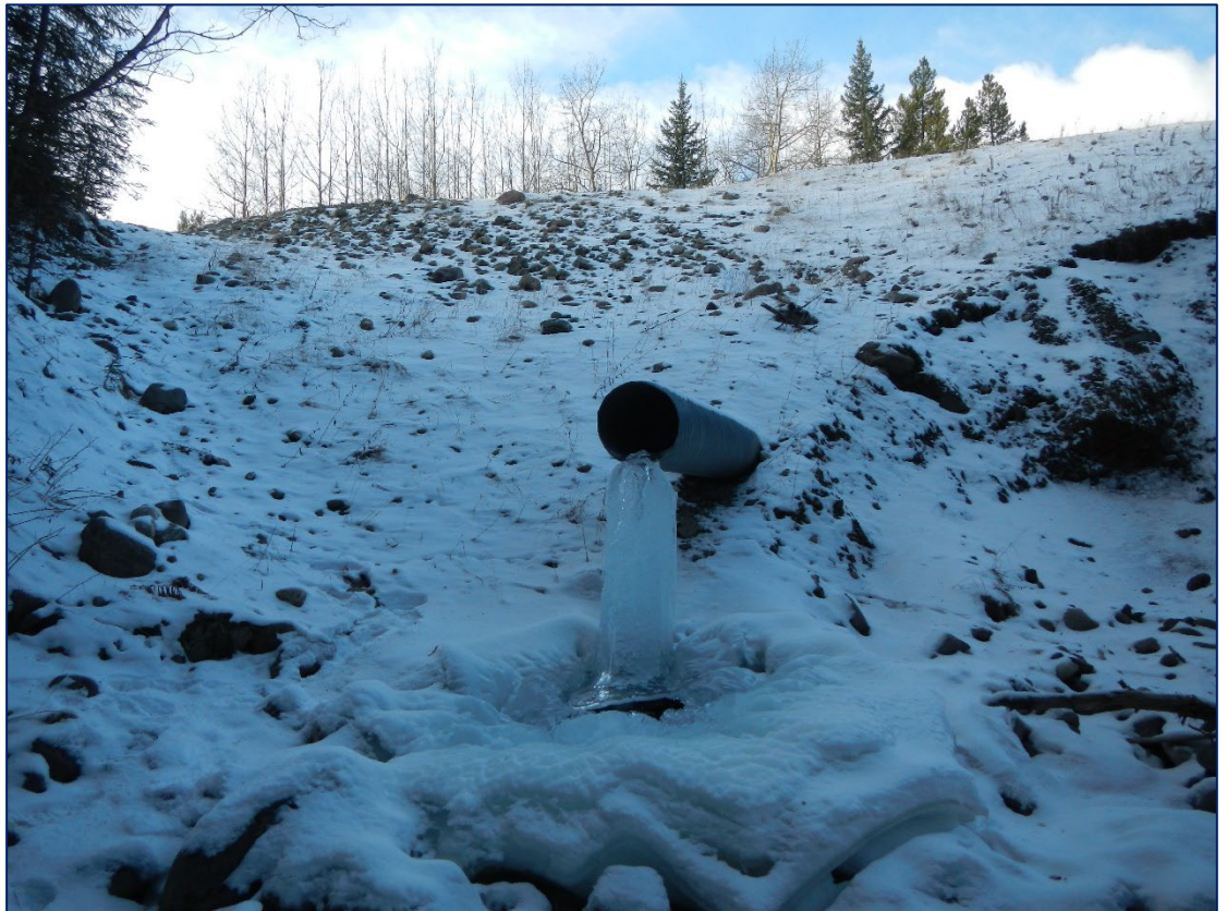
View of Downstream End.
