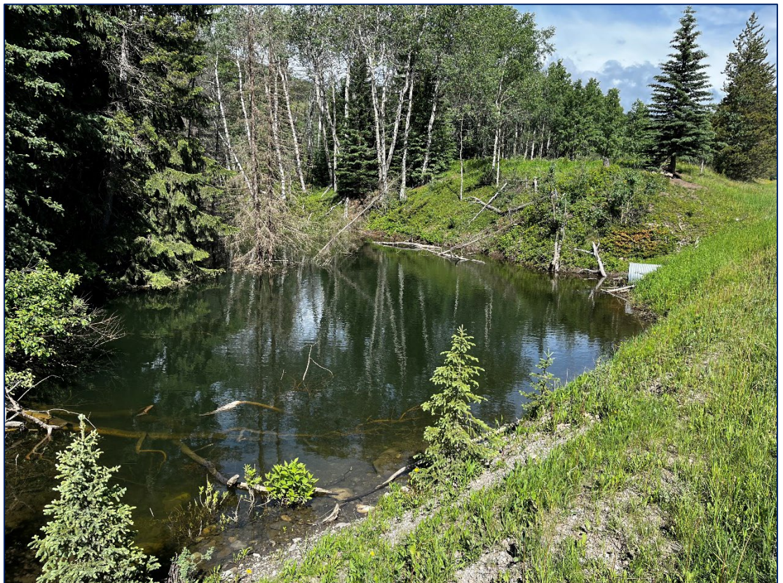
Looking Upstream from southwest corner. Water has ponded up to 7m above streambed. Ponded water is a hazard for travelling public.
