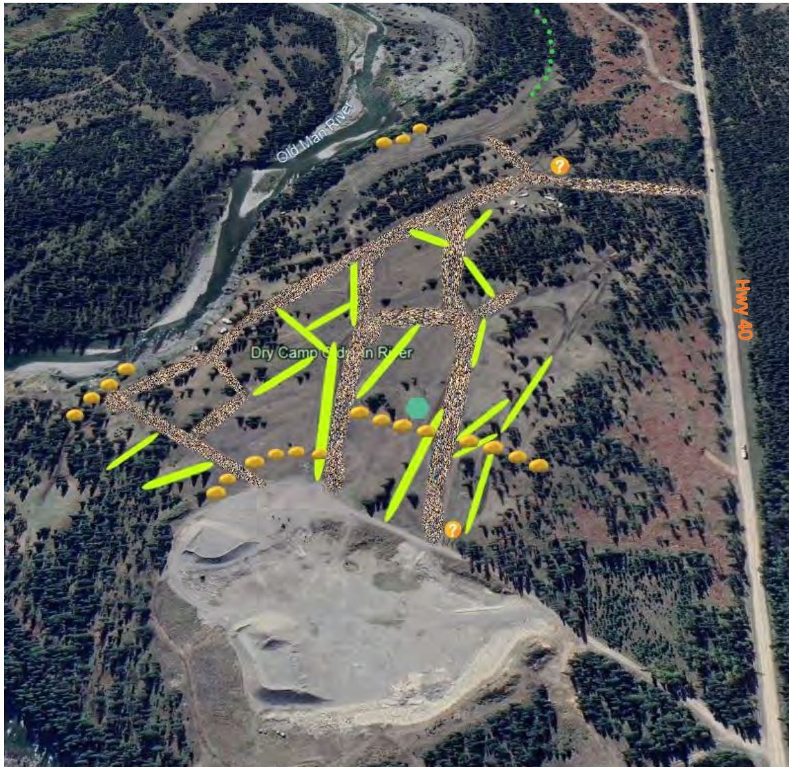
Figure 3: Dutch Flats north end: south facing direction
